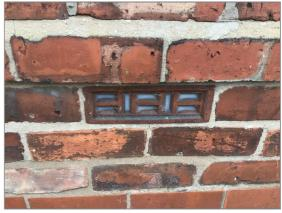
Photo - 11 Sealed cavity vents
