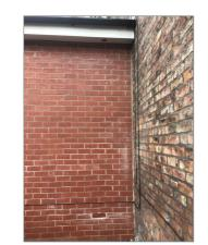
Photo - 12 Junction of rear extension, no movement
