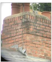
Photo - 3 Loose step flashing
