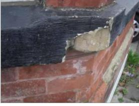
Photo - 15 Spalled window sill
