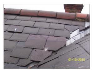
Photo - 6 Slipped slated to the rear
