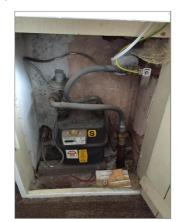
Photo - 32 Gas meter with dated lead pipes
