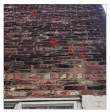
Photo - 17 Cracking over kitchen window
