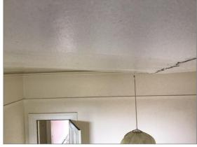
Photo - 23 Cracking and deflection to bedroom ceiling
