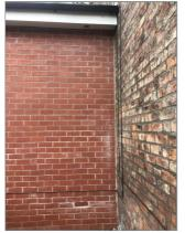
Photo - 12 Junction of rear extension, no movement
