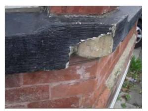
Photo - 15 Spalled window sill
