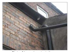
Photo - 8 Loose downpipe to the rear
