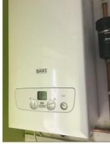
Photo - 33 Gas combination boiler
