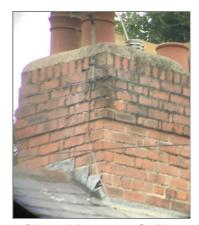
Photo - 3 Loose step flashing
