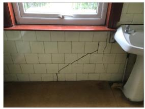
Photo - 25 Cracking to bathroom tiles
