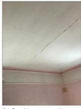
Photo - 24 Cracking to reception room ceiling
