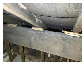
Photo - 21 Purlin has been packed to support rafters.
