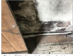
Photo - 26 Mould growth the gable wall not damp
