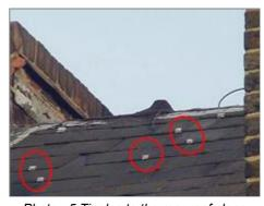
Photo - 5 Tingles to the rear roof slope
