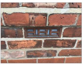
Photo - 11 Sealed cavity vents
