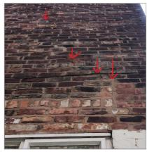
Photo - 17 Cracking over kitchen window
