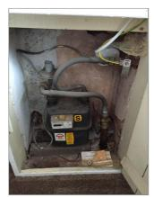
Photo - 32 Gas meter with dated lead pipes
