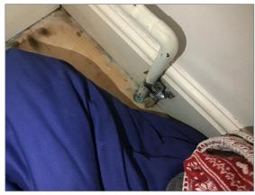
Photo - 19 Bonding to gas pipe
