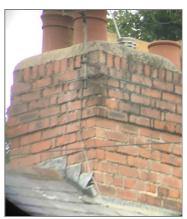
Photo - 3 Loose step flashing
