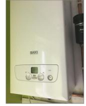
Photo - 33 Gas combination boiler
