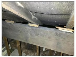
Photo - 21 Purlin has been packed to support rafters.
