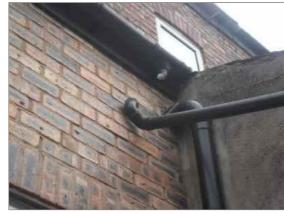
Photo - 8 Loose downpipe to the rear
