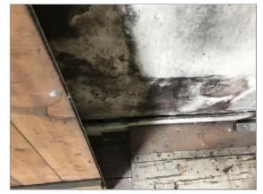
Photo - 26 Mould growth the gable wall not damp
