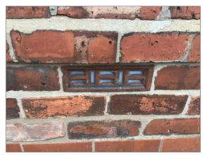
Photo - 11 Sealed cavity vents
