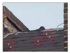
Photo - 5 Tingles to the rear roof slope
