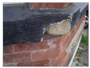
Photo - 15 Spalled window sill
