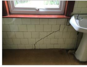
Photo - 25 Cracking to bathroom tiles
