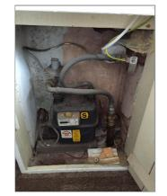
Photo - 32 Gas meter with dated lead pipes
