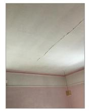
Photo - 24 Cracking to reception room ceiling
