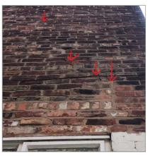
Photo - 17 Cracking over kitchen window
