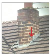
Photo - 3 Missing flashing
