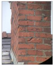
Photo - 2 Spalling brickwork
