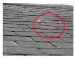
Photo - 5 Metal clips used to repair covering
