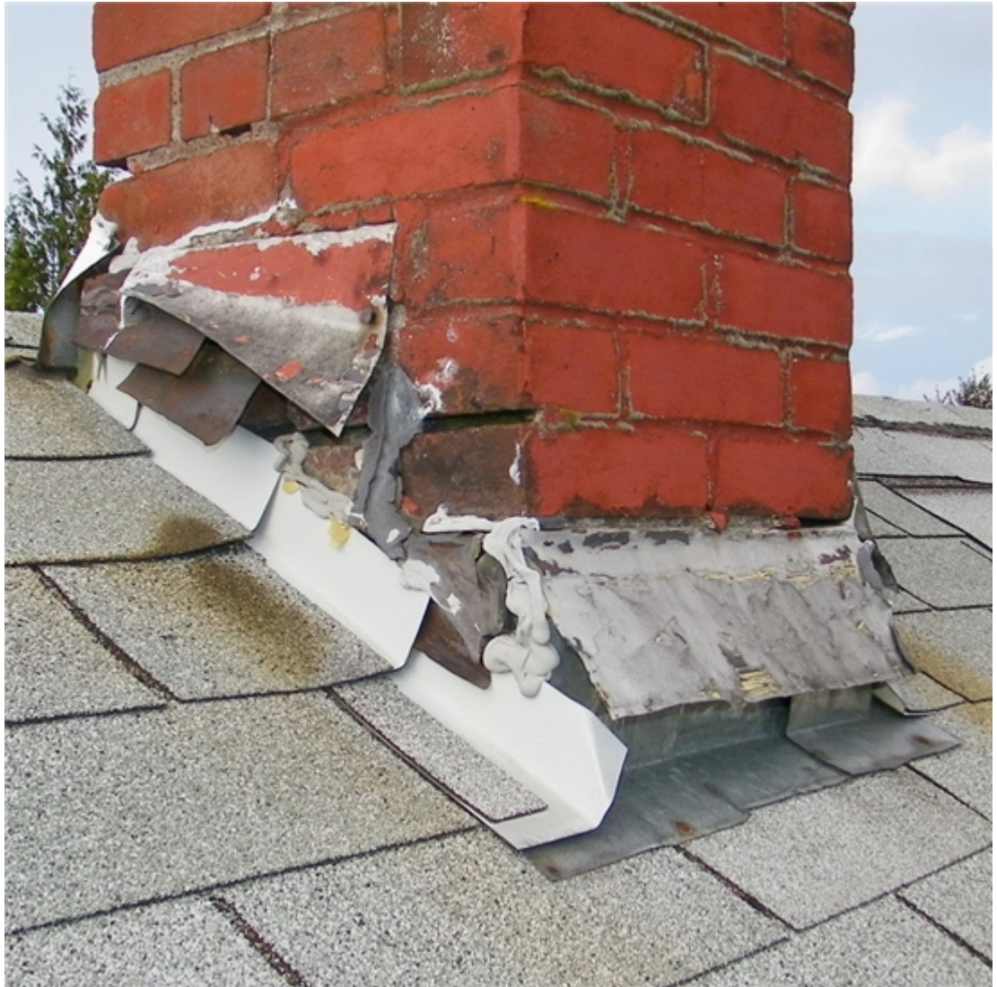
Poor flashing to the rear stack
