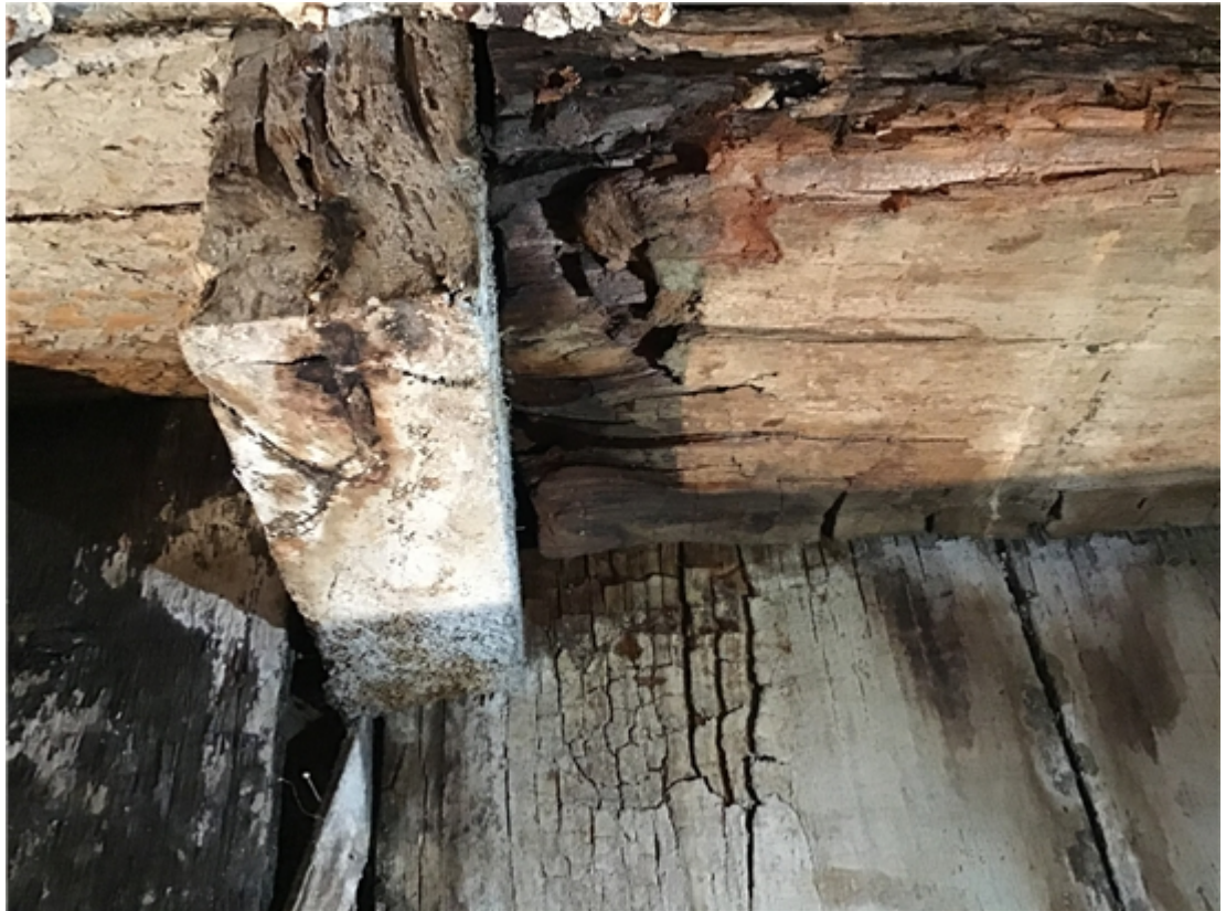
Isolated rot around chimney breast
