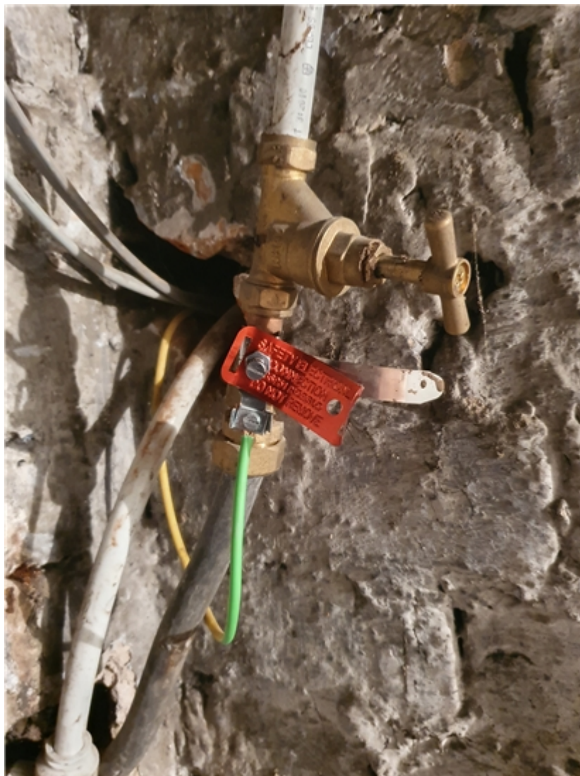
G3: Lead water supply pipe.
